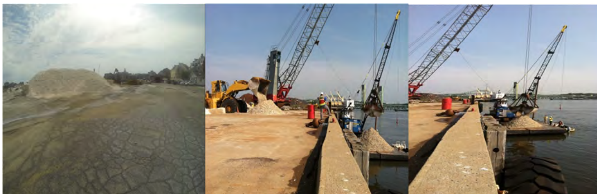
Fig 3. Staging operations at Granite State Minerals, Portsmouth, NH
