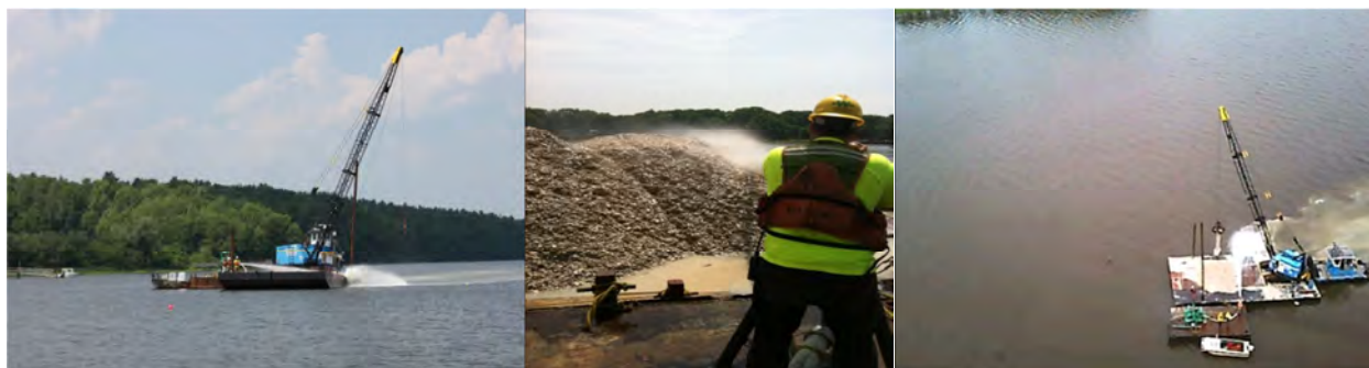
Fig 4. Shell deployment from barge using diesel pump and fire hose assembly
