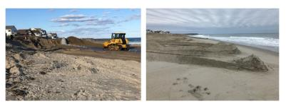
Sand being pumped on the beach north of SB02 on Oct 16, 2019 (left). The sand is immediately spread by bulldozers (right) and over time by natural processes.
